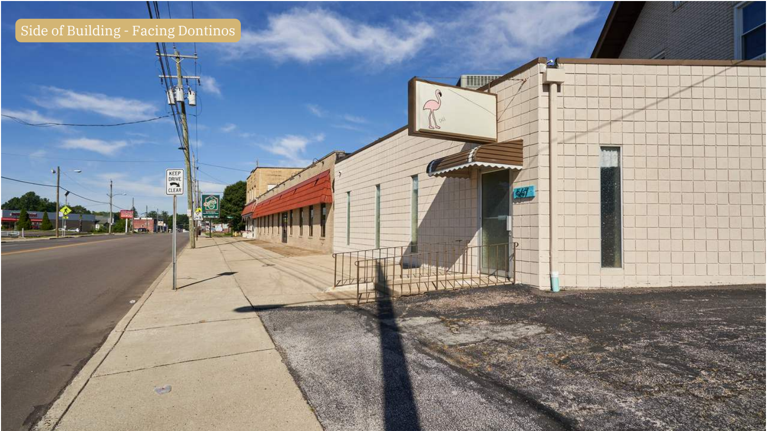
Front Building - E Cuyahoga Falls Ave
