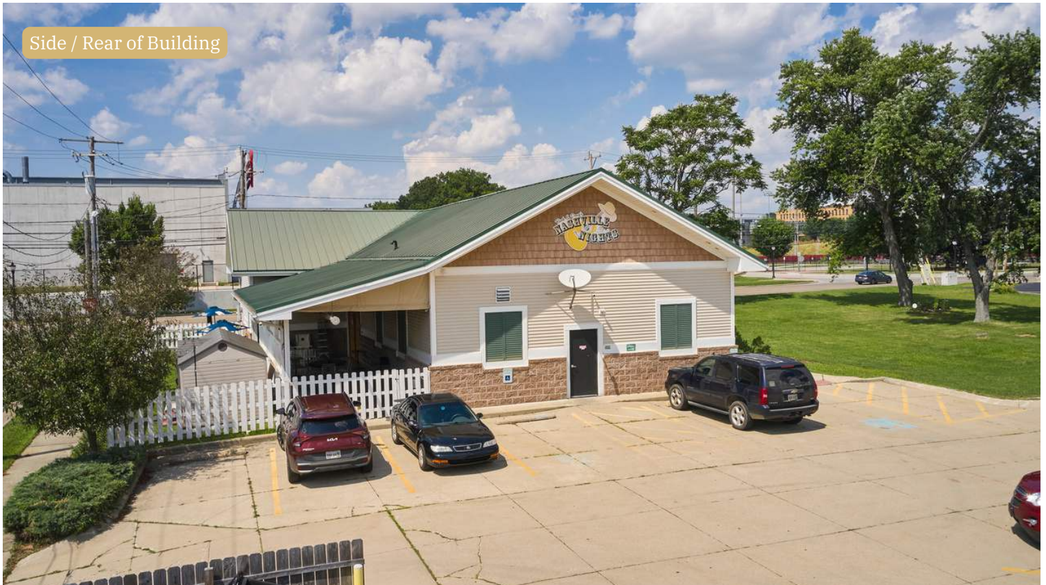
Front Building /Side of Building
